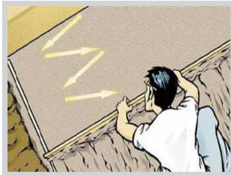
vlakmaken zand/splitbed
